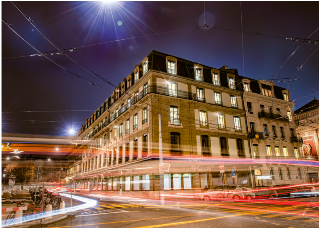
The Bank's headquarters on the Boulevard du Théâtre in Geneva.
